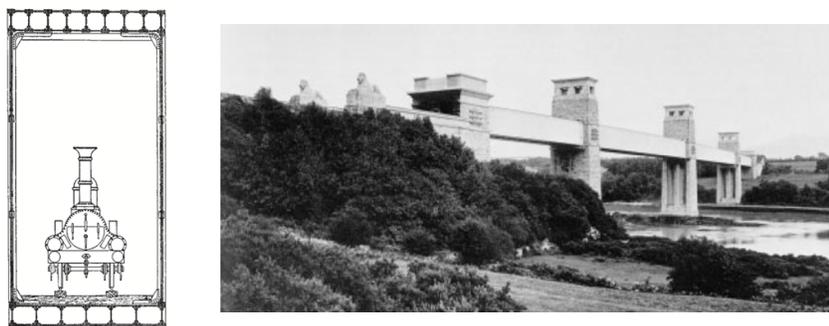
**Fig. 2.1.** The innovative Britannia bridge over the Menai Strait by Stephenson. The original structure stood in this form until 1970, when the bridge was damaged in fire and replaced. The locomotives ran through metal tubes of multi-cellular cross section.
